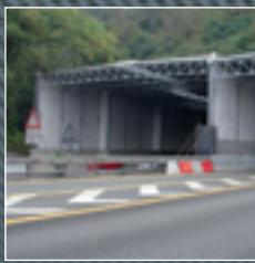
**CE marked panels according to EN 14388 norm (road noise reduction devices)**
